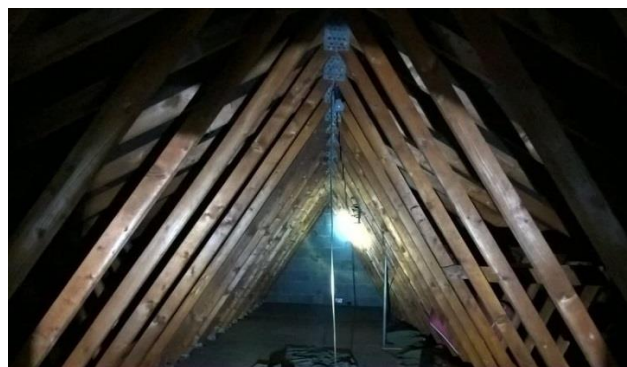
Plate 4.11: Loft Space of No. 80 Tatenhill Lane.
