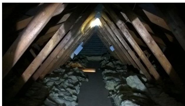
Plate 4.6: Loft Space of No. 78 Tatenhill Lane.
