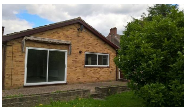
Plate 4.2: South-western Elevation of No. 78 Tatenhill Lane.
